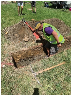
(c) Footings dug by hand
