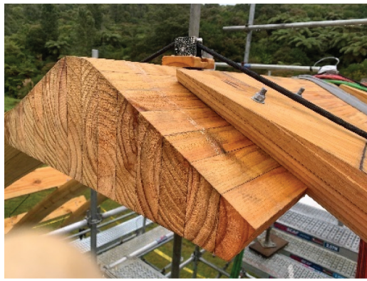
(a) High-load exit box mounted on ridge beam (tāhuhu)
