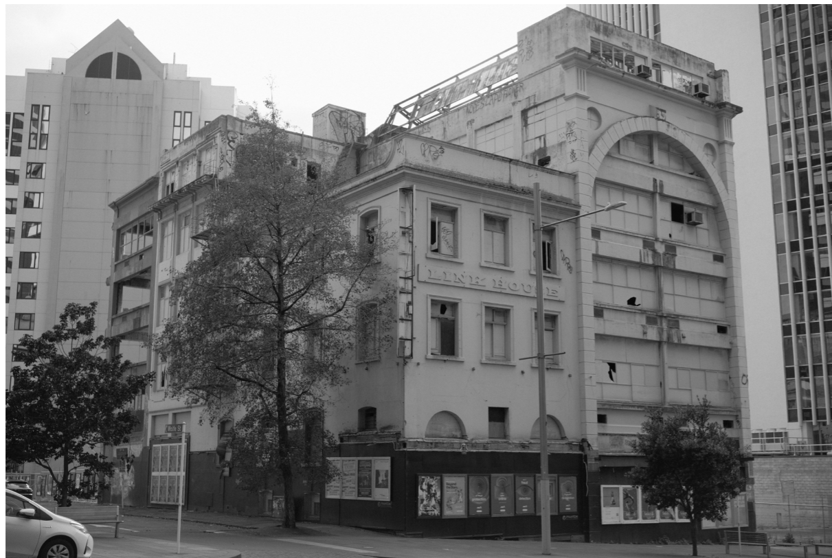
Figure 27. Image of Yates Buildings site, by Author.
