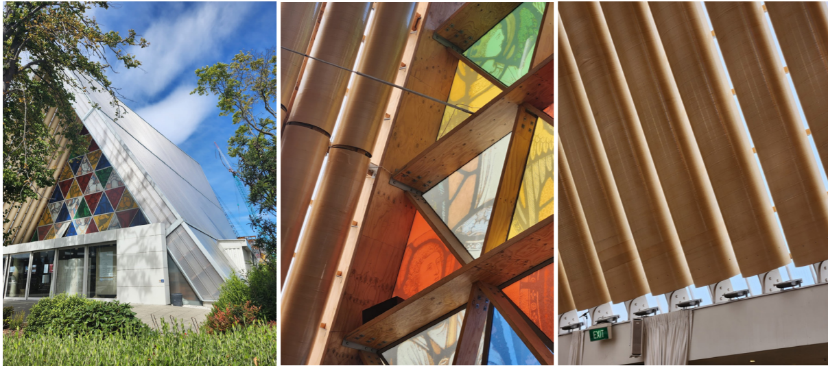
Figure 14. Image of Transitional Cathedral Exterior, by Author. Figure 15. Image of Transitional Cathedral interior window, by Author. Figure 16. Image of Transitional Cathedral structure, by Author.
