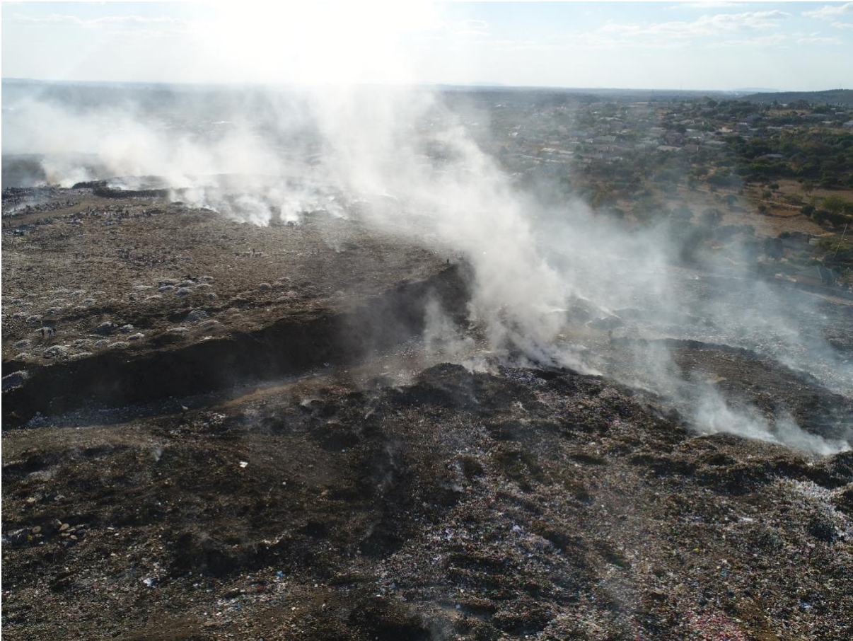
Figure 5:20: Smoke Plumes from subsurface fires at Chunga landfill resulting from multiple fire focal points across the landfill. The Plume blows primarily west to south west affecting residents of surrounding communities.
