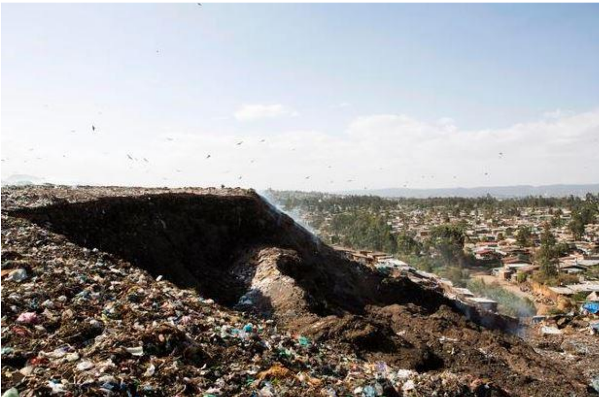
Figure 6:1: The mountain of waste at Koshe Landfill in Addis Ababa that collapsed due to excessive dumping and slope failure (Raviteja & MunwarBasha, 2017)
