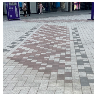
Concrete Tile Flooring at Commercial Bay, Auckland, 2022
