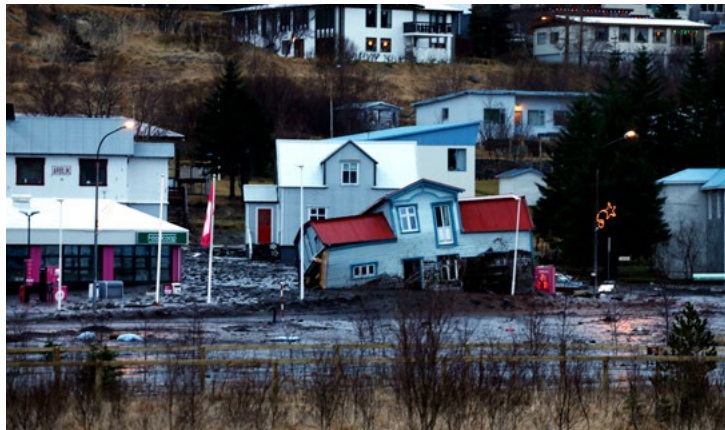
Fig 116. Seyðisfjörður Landslide 2020, Eggert. Jóhannesson for MBL. https://www.mbl.is Seyðisfjörður 2020. Here you see the house Breiðablik in front of the gas station. Its original foundation is above the far left house.
