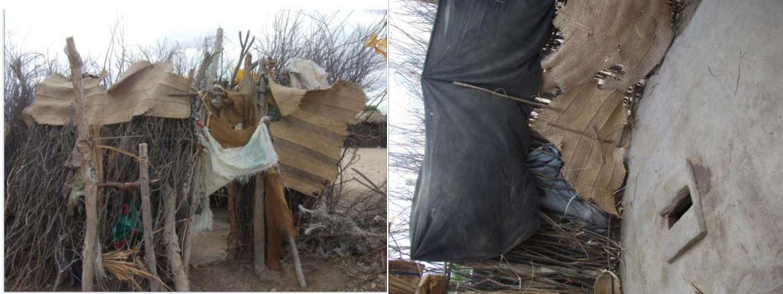
Figure 12: A Household latrine made from locally available materials with images that represent view from outside and inside (note the small openings in picture 2 that can compromise privacy).
