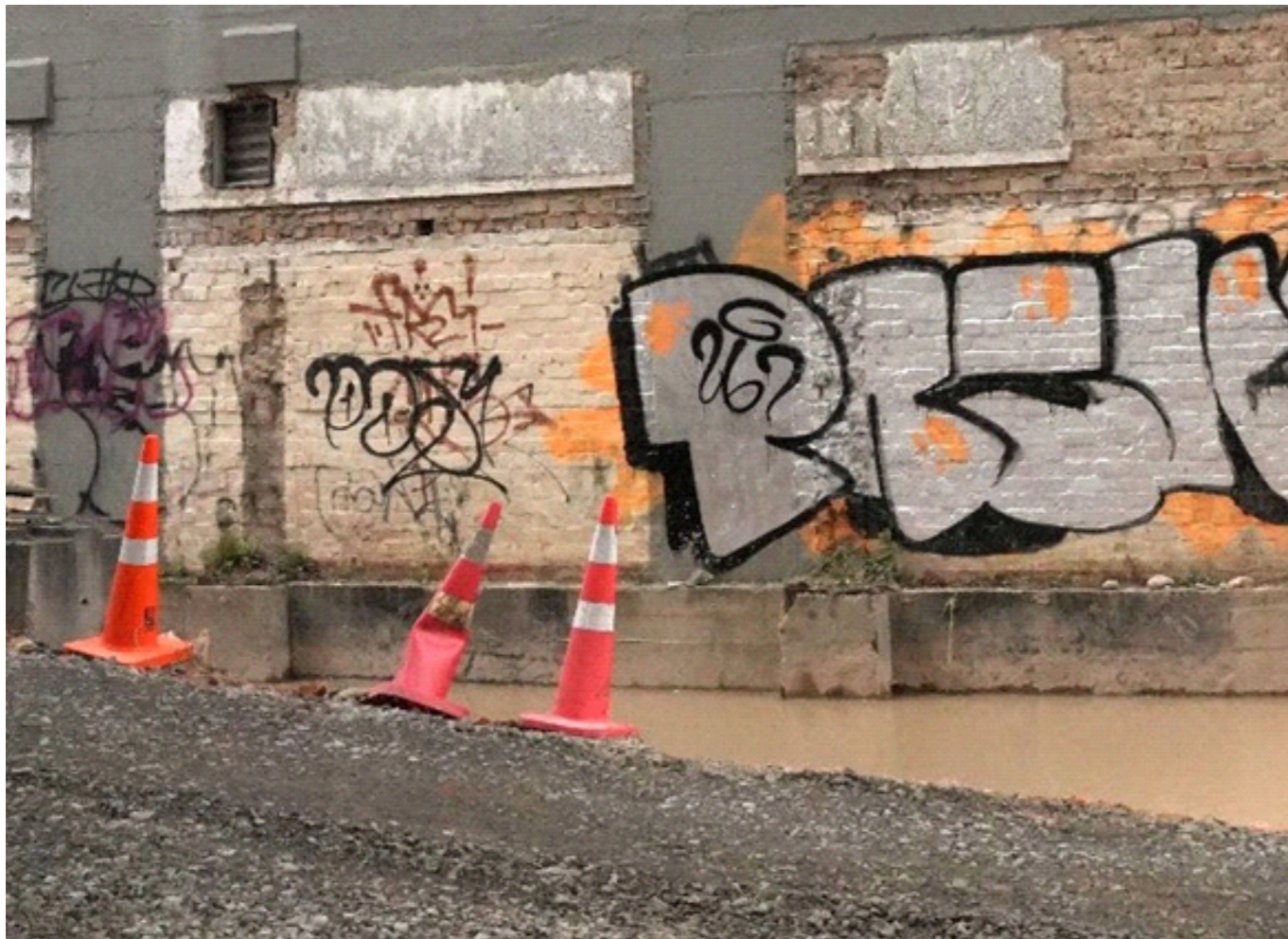
Figure 13. Photo of flooded site of St James Theatre (2025).
