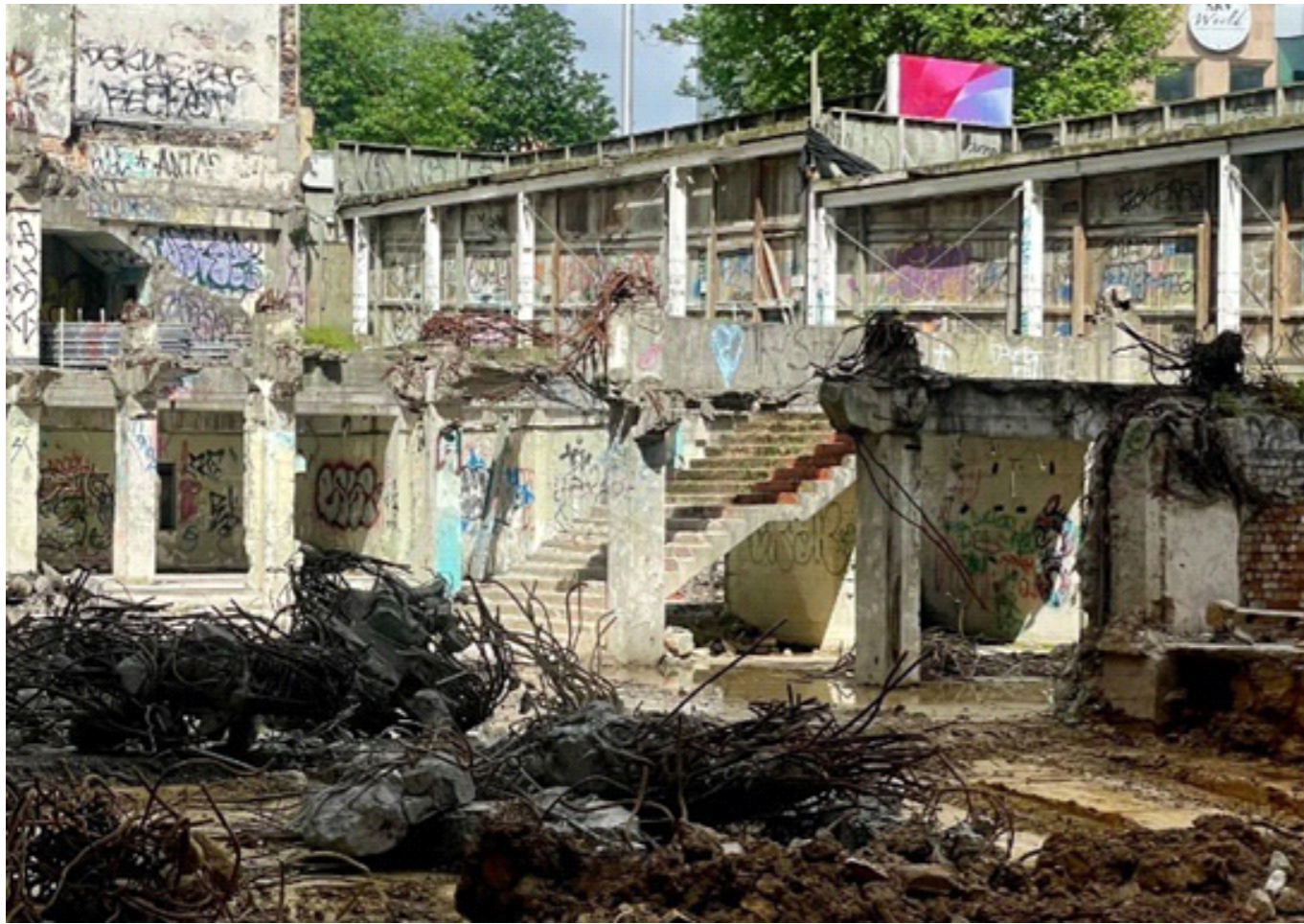
Figure 12. Photo of construction site in St James Theatre Site (2025).
