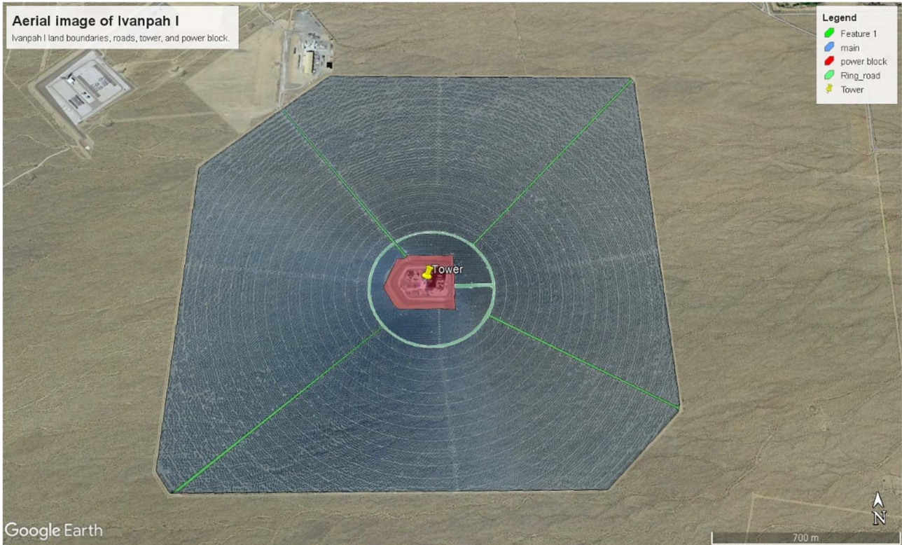
Fig. 7 Aerial image of Ivanpah I, CA, USA
