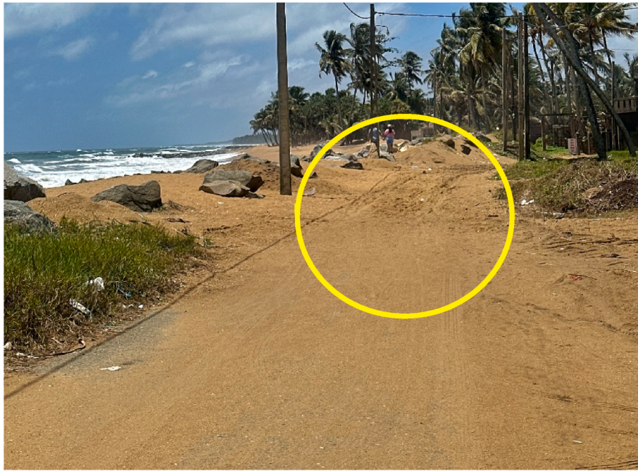
Fig. 4. Example of infrastructure impacts associated with sand accumulation at Calido Beach. Photograph showing sand deposition on access roads and within drainage channels following coastal change and mitigation efforts. Sand accumulation has reduced accessibility and disrupted drainage function in the study area. Note: Image captured during field visit in 2025.
