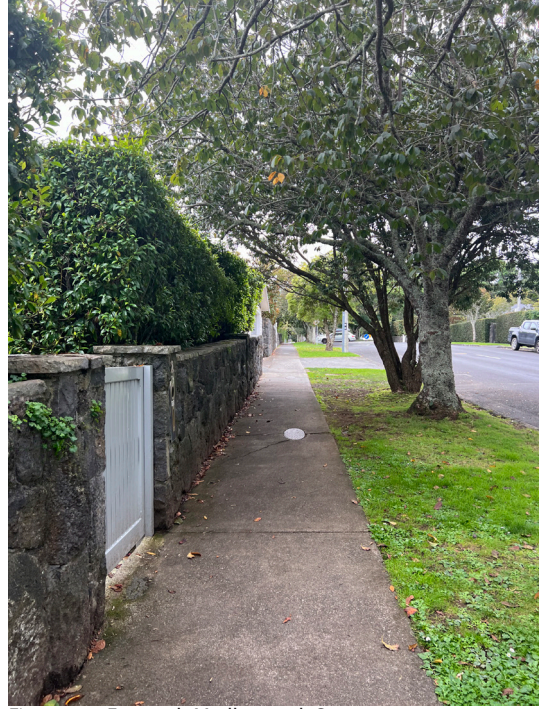
Figure 69 - Footpath Marlborough Street
