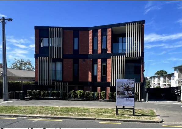
Figure 13 - View Road Apartments
