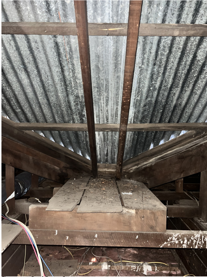
Figure 118 - Roof Gutter Support
