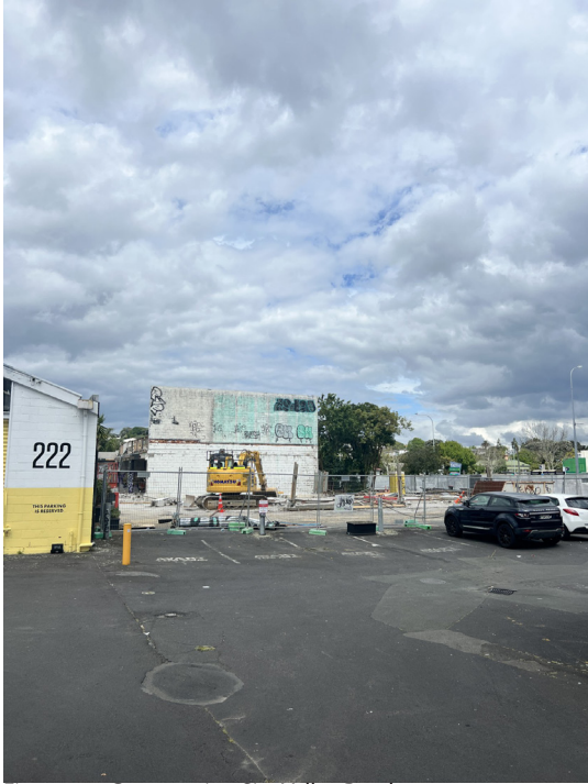
Figure 74 - Construction Site Valley Road
