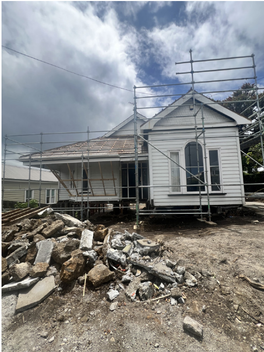
Figure 70 - Paice Ave Villa
