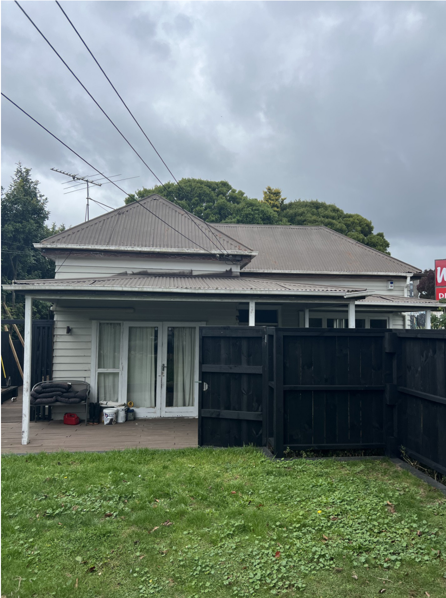
Figure 107 - Exterior of the Existing Building
