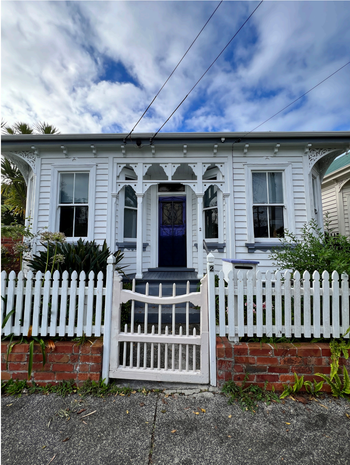
Figure 98 – Visible Building Entrance Close to the Street
