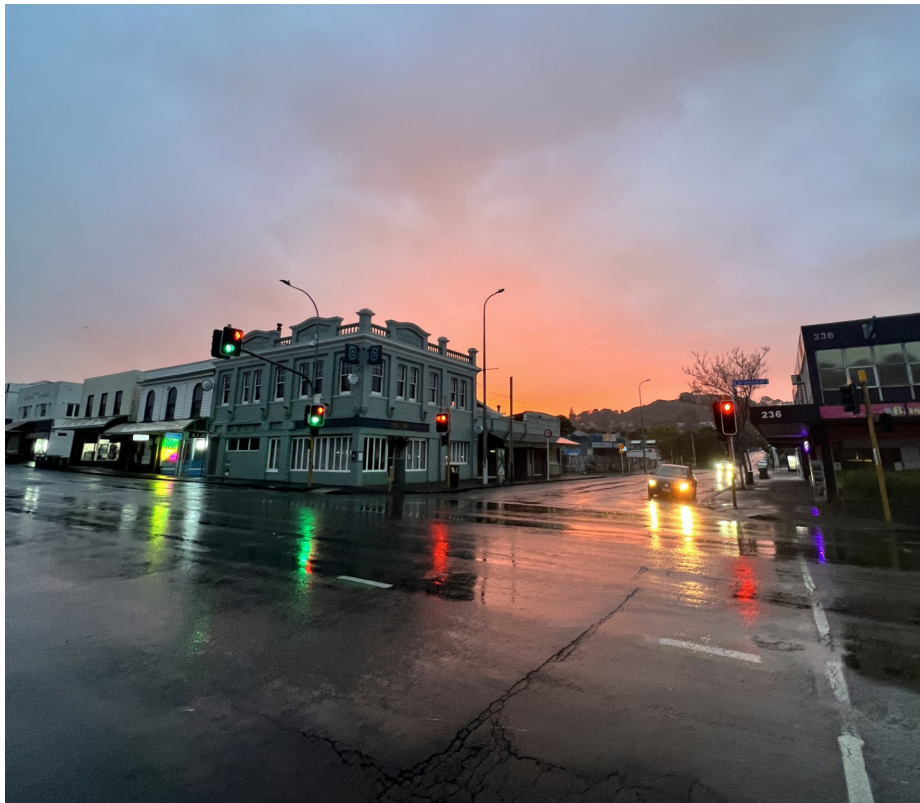
Figure 59 - The Corner of Dominion and Vally Road
