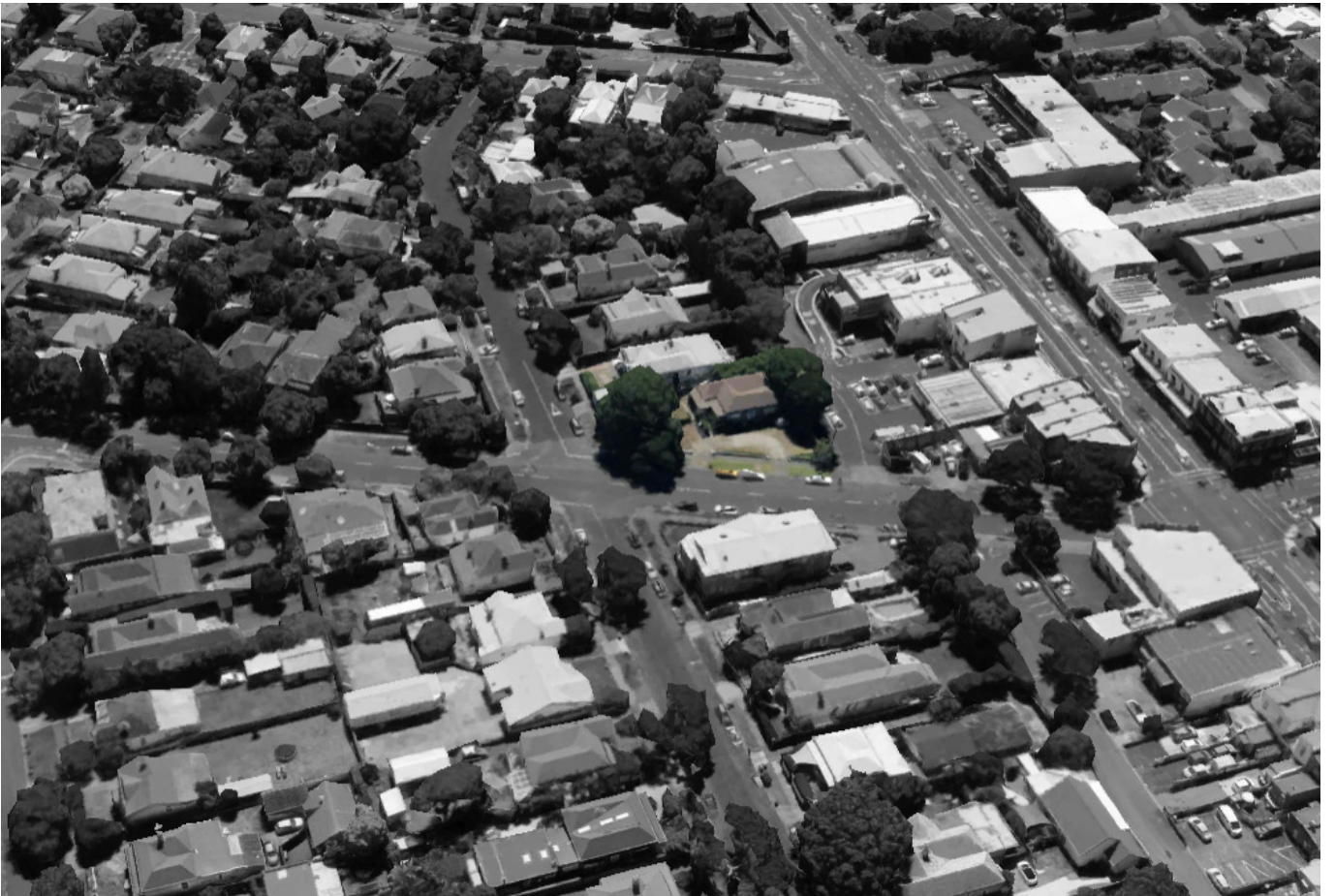
Figure 102 - Walters Road Site (Google Earth, n.d.)
