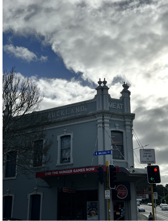
Figure 73 - Auckland Meat Building Dominion Road
