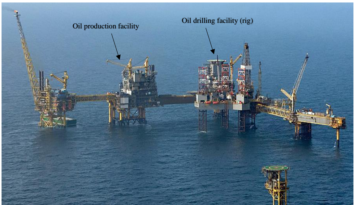
Figure 1.2: Typical set up of drilling and production facility (source- http://argoflares.com/wp-content/uploads/2012/01/Offshore-Complex.jpg )
