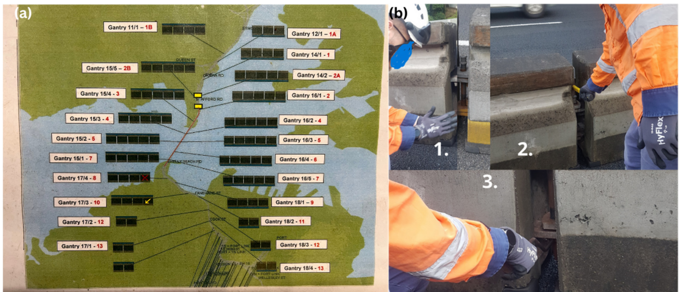
Figure 2. The scale of the challenges for manual inspection and fixing of the metal pin: (a) various locations of movable concrete barriers on and around the Auckland Harbour Bridge; (b) finding an unsafe pin and fixing it manually.
