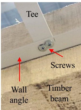
Figure 14. Tee connected to wall angle using double screws at the fixed end.
