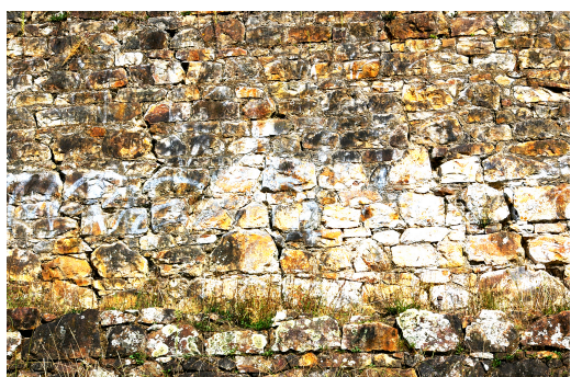
Figure 12. Farquhar, A. (2010). Karangahake Gorge [Digital photograph].
