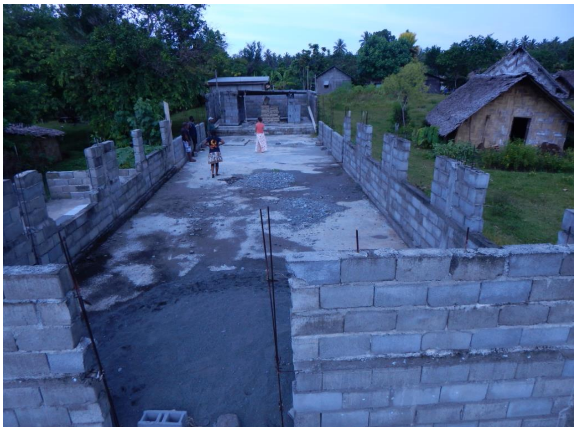
Figure 12: Ipayato community build a community evacuation centre
