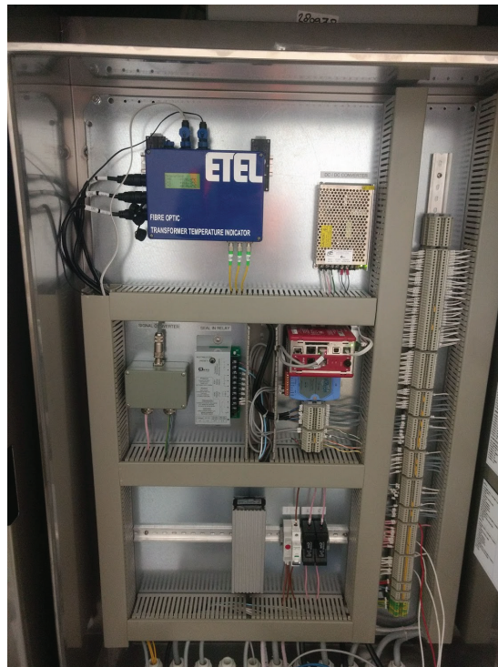
Figure 6.7: Physical Implementation of Marshalling Box in Fig. 6.5.
