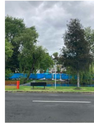
On-going construction at Portland Reserve. 05 November 2021, 4.15pm
