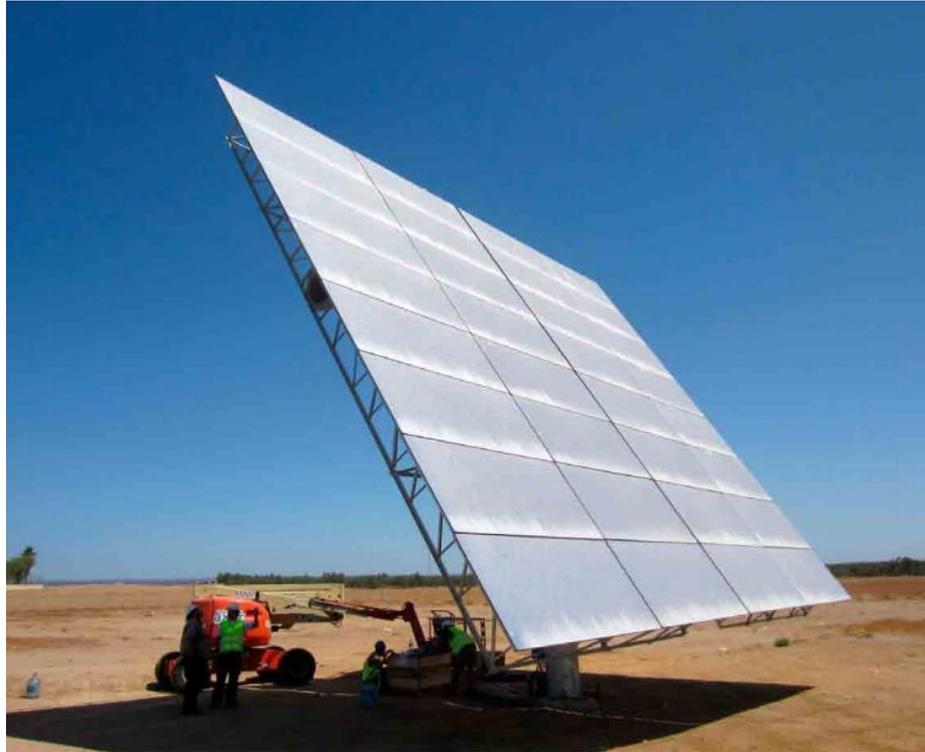
*Figure 14: Abengoa ASUP 140 heliostat*
