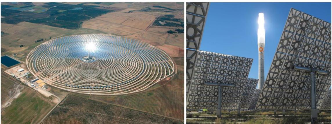
*Figure 7: Heliostat field in solar central tower power plant*
