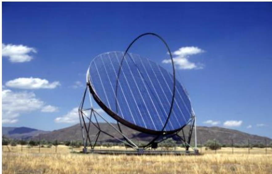
***Figure 10: ASM-150 heliostat***
