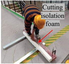
Figure 17. Preparation of isolation foam.
