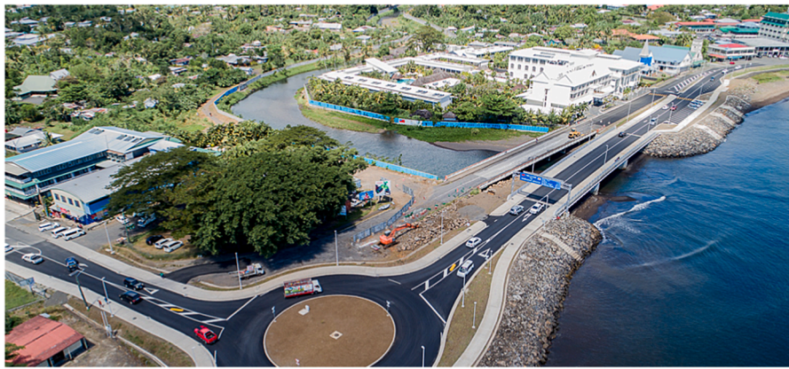
Fig. 5. The Vaisigano Bridge. Image by Samoa Observer, 2020.
