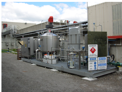
(a) TERAX stage 1: 2000L anaerobic fermentation unit
