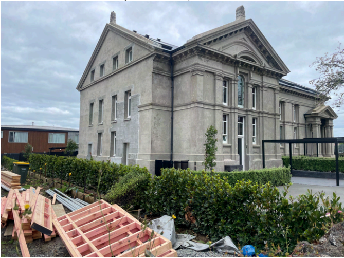
South Side of the Church with Newly Added Windows, 2025
