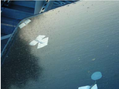
Figure 7. Condensation on collector
