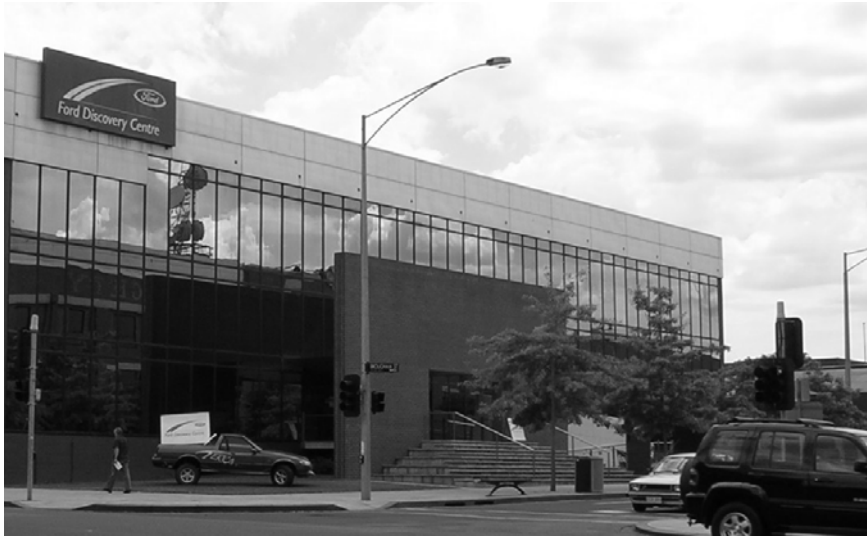
Figure 1: Eastern glazed facade of office building
