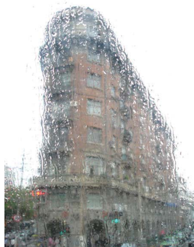
Fig. 3.3 Lu 2006 Photograph of window
