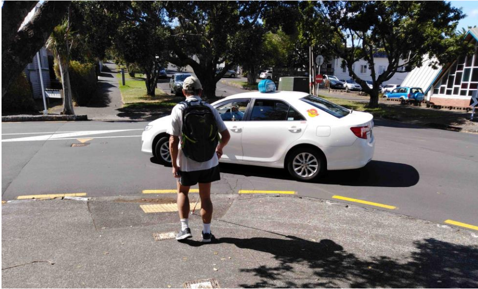
Figure 21: Informal crossing of a side street with tactile pavers and an open curb; photo taken by TB, walking with Ollie
