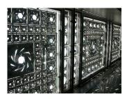
Fig. 11 Jean Nouvel's Institute du Monde d''Arabe has an intricate facade that modulates light to the interior using shutters that open and close like a camera lens.
