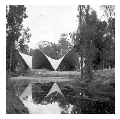
Fig. 14 Lightweight concrete parabolic roof structure designed by Felix Candella.
