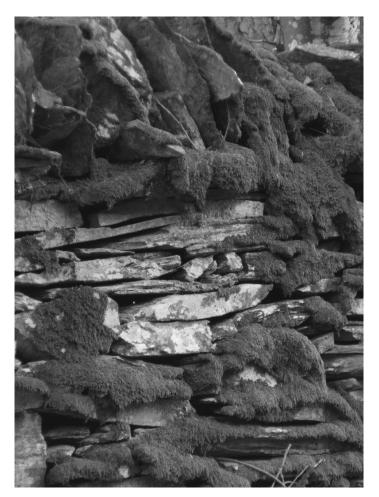
Fig. I The most sustainable approaches to building use materials that are locally available, which can transform over time through weathering without detriment to performance as in this example of a dry stone wall covered in moss.
