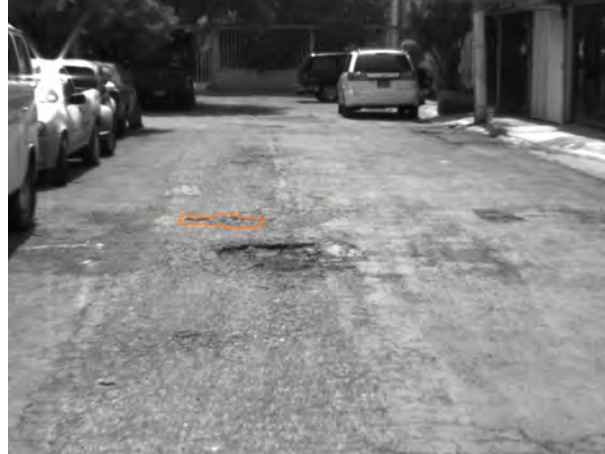
Figure 5.17: Pothole candidate marked with orange colour is hard to identify for annotation.
