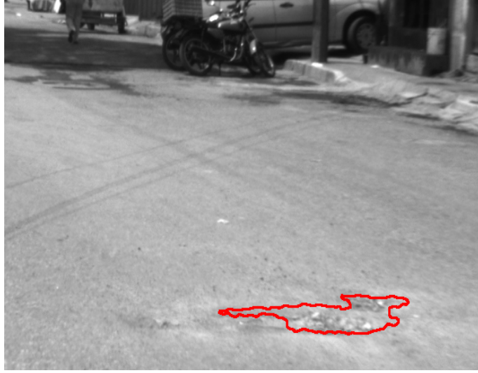
Figure 4.22: Outline of potholes identified from a multi-frame DEM, after projecting the valley cells into image domain and triangulating the vertices using alpha shapes.
