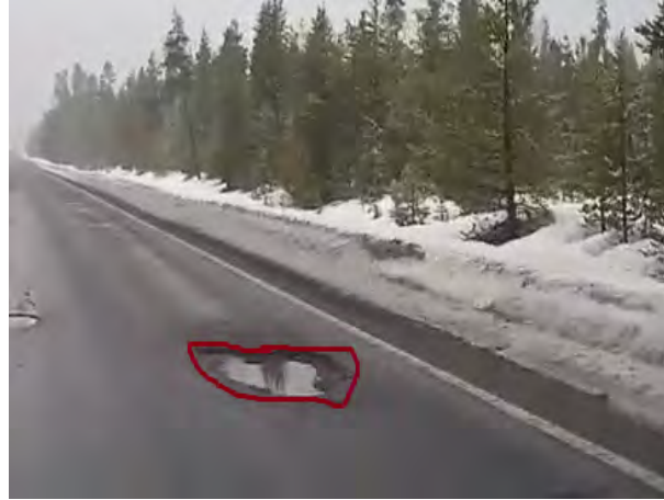
Figure 5.11: Pothole marked in red colour presents a very complex situation as it is filled with water and shadow of a tree.
