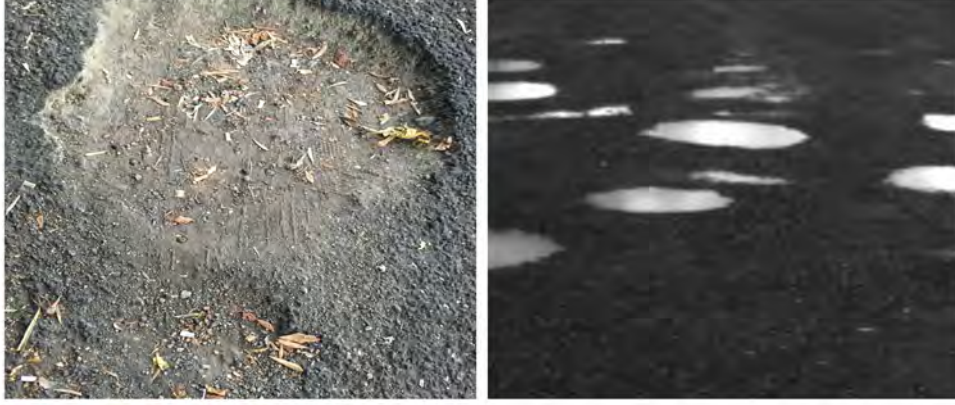
Figure 1.2: Dried leafy pothole on the left, and water filled pothole on the right, showing different intensities of light
