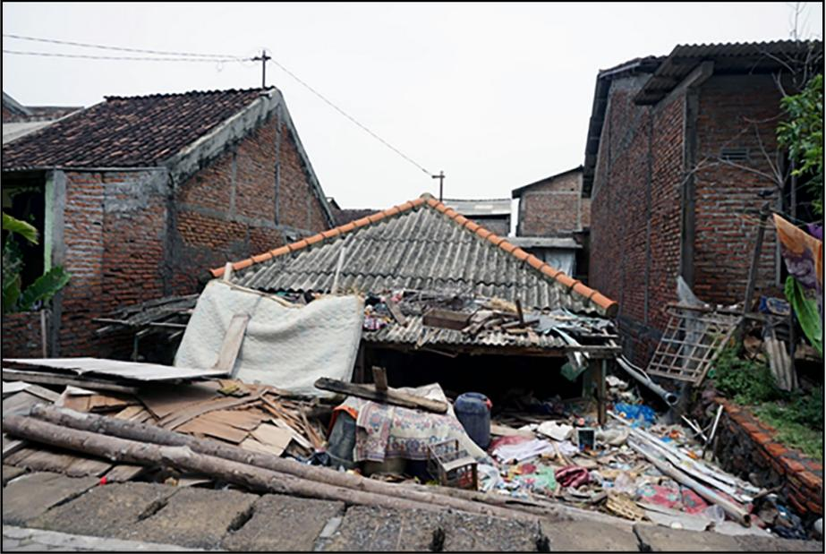
**Figure 3: Houses damaged and abandoned due to rob floods and land subsidence in Tambak Lorok fishing village, Semarang.**
